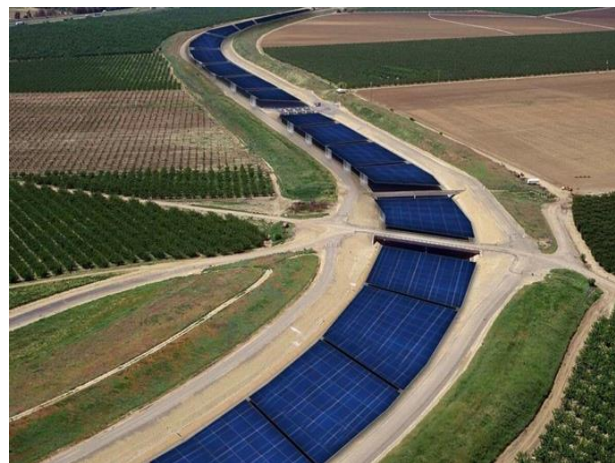
Figure 6. Solar Panels Mounted On Irrigation Canals
